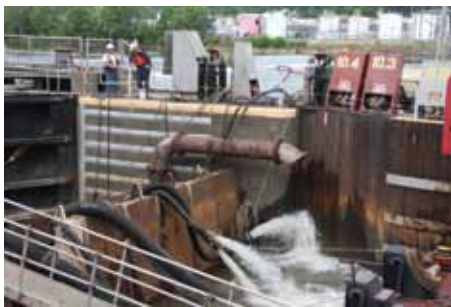
Pittsburgh District maintenance workers pump out the auxiliary lock chamber ahead of scheduled repairs to the aging, pre-World War 1 facility. The Corps planned to remove the structure in 2004.
